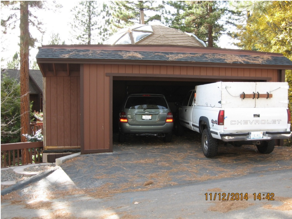
Photograph of the enclosed carport with the two foot extension
